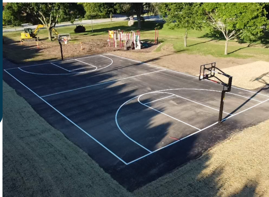
Columbia Park Basketball Court and Playground Install
