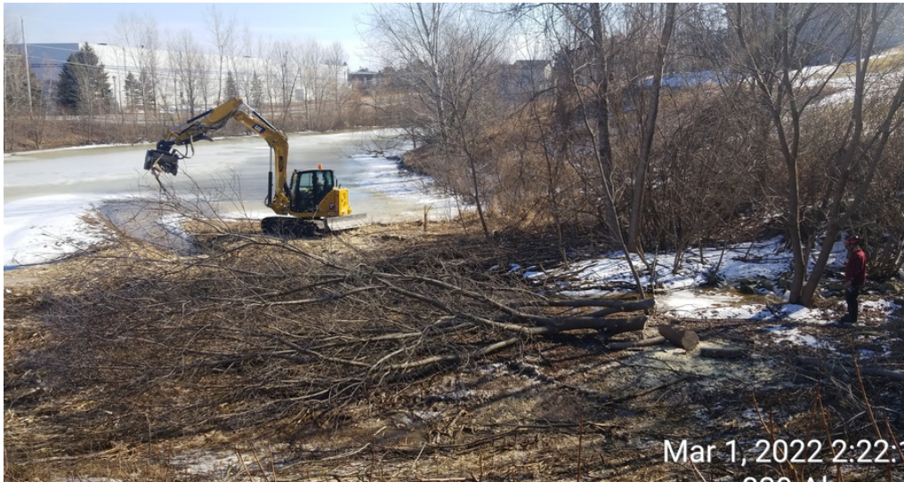
Retention Pond Maintenance
