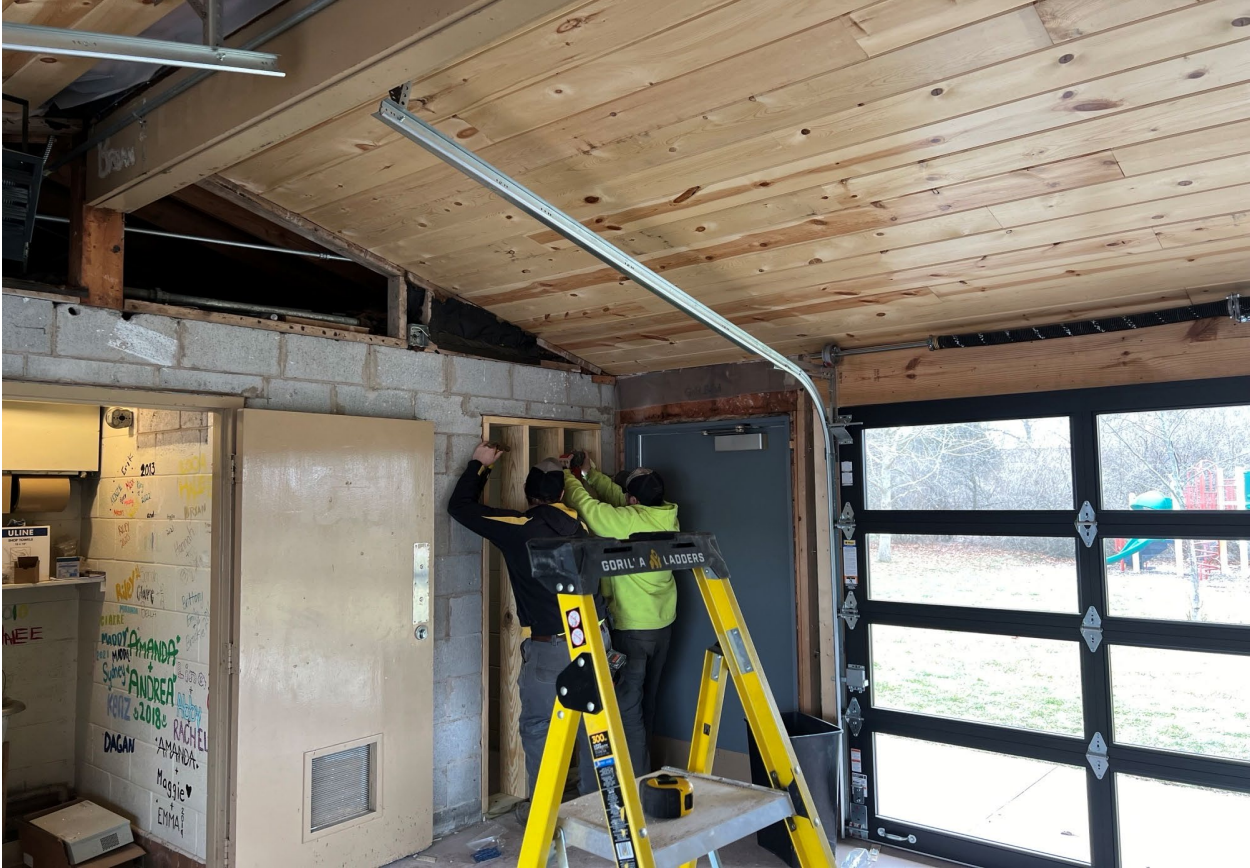
Kolbach Park Shelter Remodel
