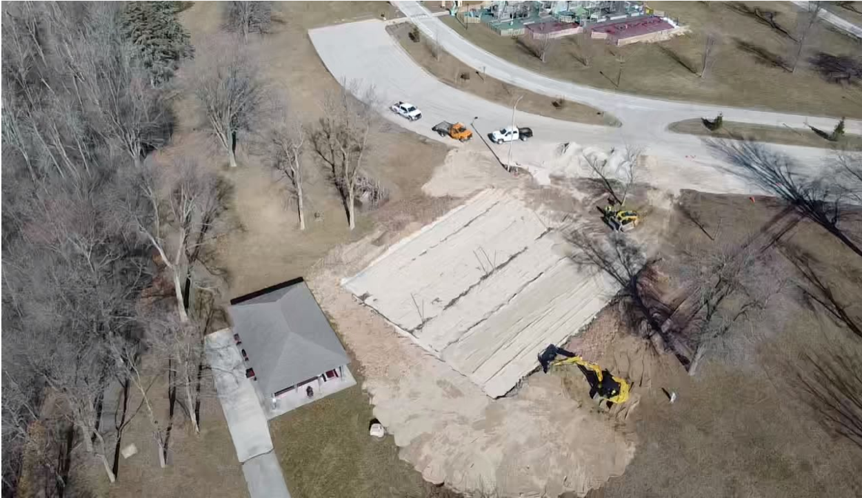
Volleyball Court Construction
