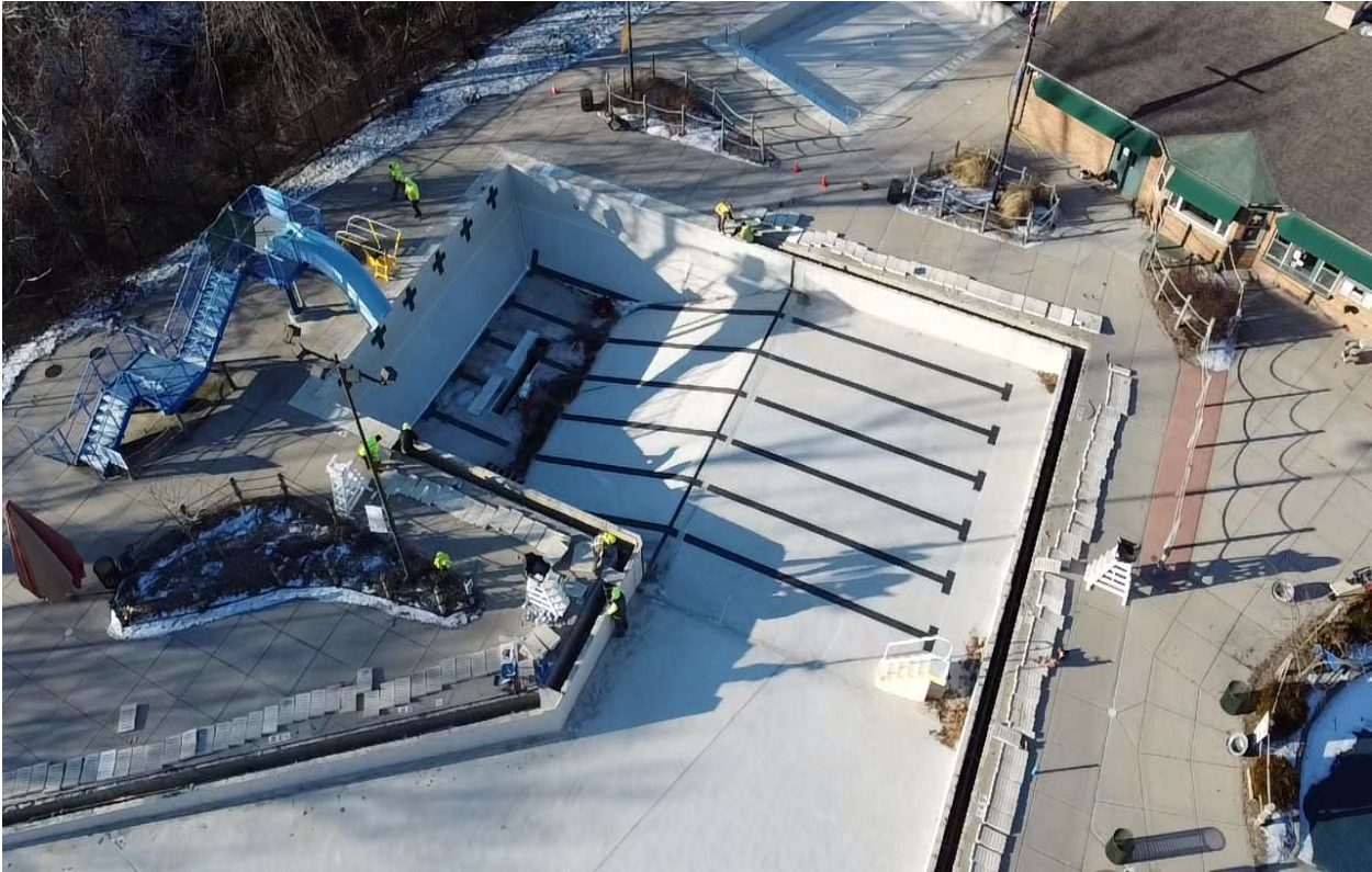
Gutter Stone Removal
