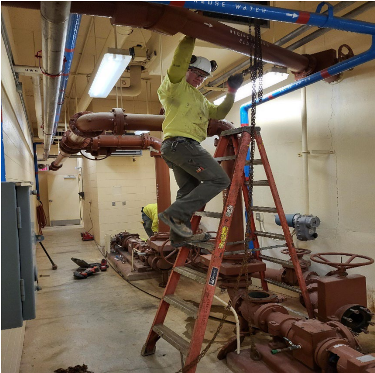
Figure 1 - Demo of pumps and piping
