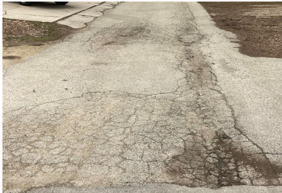
Figure 1: Alley Between Sherman and Lincoln looking south
