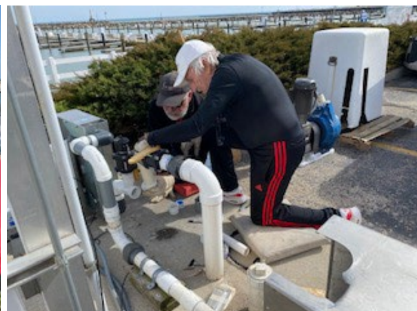
The Dennis' installing the piping for the new pump
