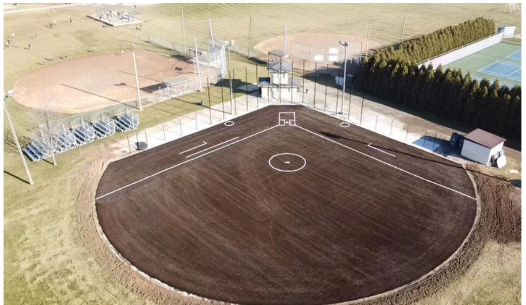
Municipal Ballfield Improvement
