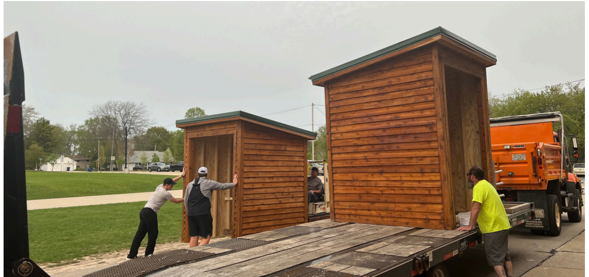
Restroom Shelter Project
