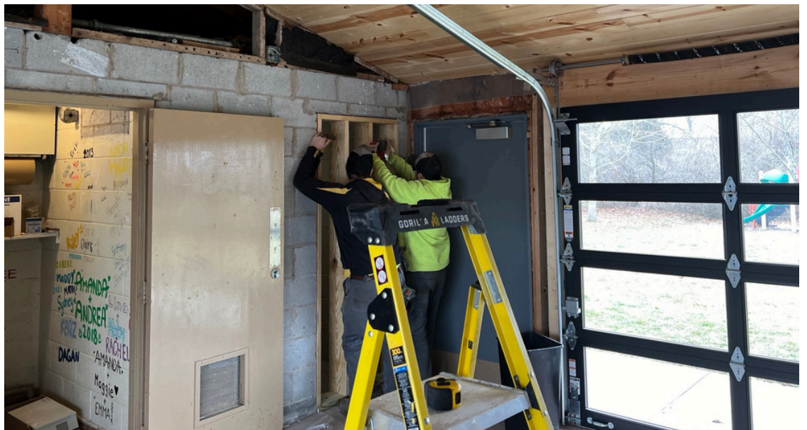
Kolbach Shelter Remodel
