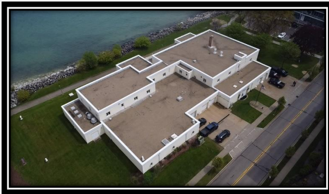
Port Washington Water Filtration Plant – 2024
