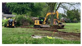
The Streets Division removing the concrete swale and installing drain tile in Kolbach park in preparation for adding an asphalt path from Jefferson St to the pickle ball courts. The Streets division also dug the rain garden in Kolbach Park off W Whitefish Rd.
