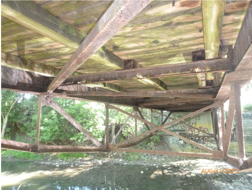
Photo 3. Cross bracing
