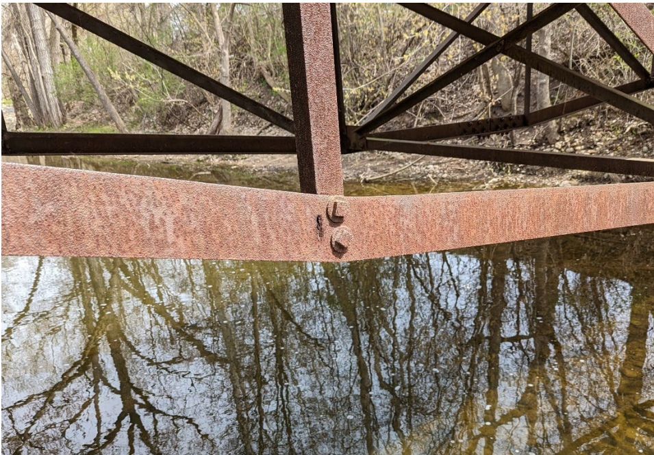
Photo 6. Lower arch connection 1 st from the west
