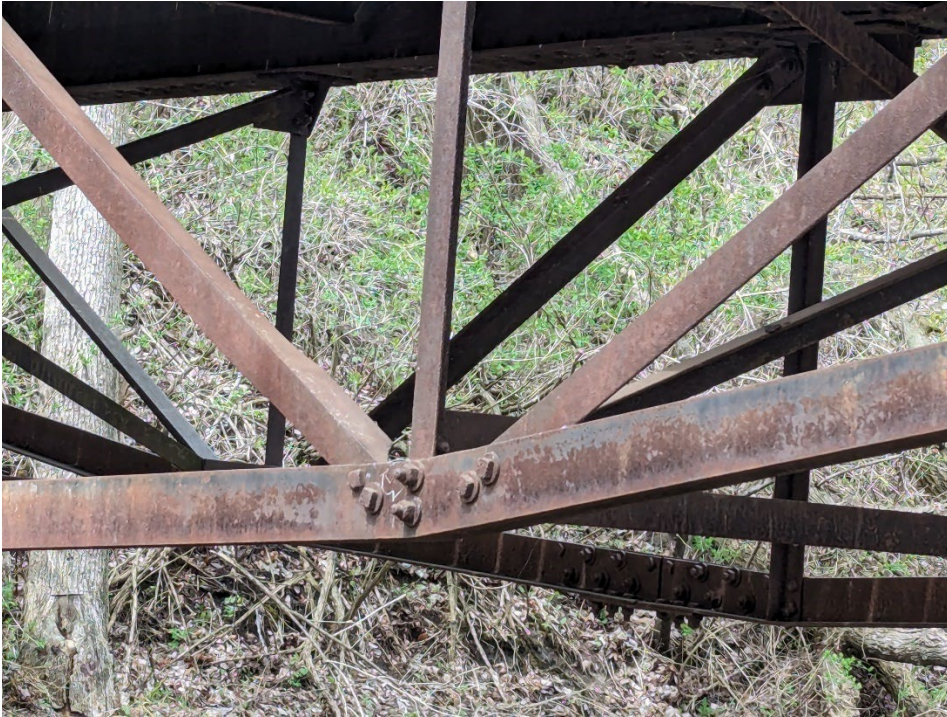
Photo 7. Lower arch connection 2 nd from the west
