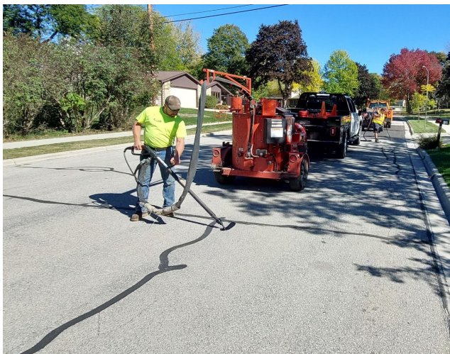
2Traditional Crack Filling Operation
