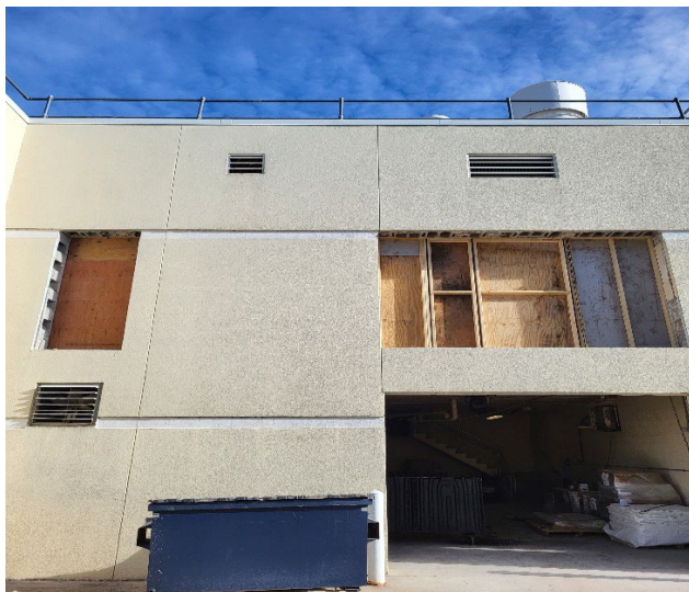
Figure 1- New second story door openings for headworks building.
