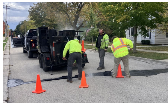
(Applying Mastic to Large Cracks)
